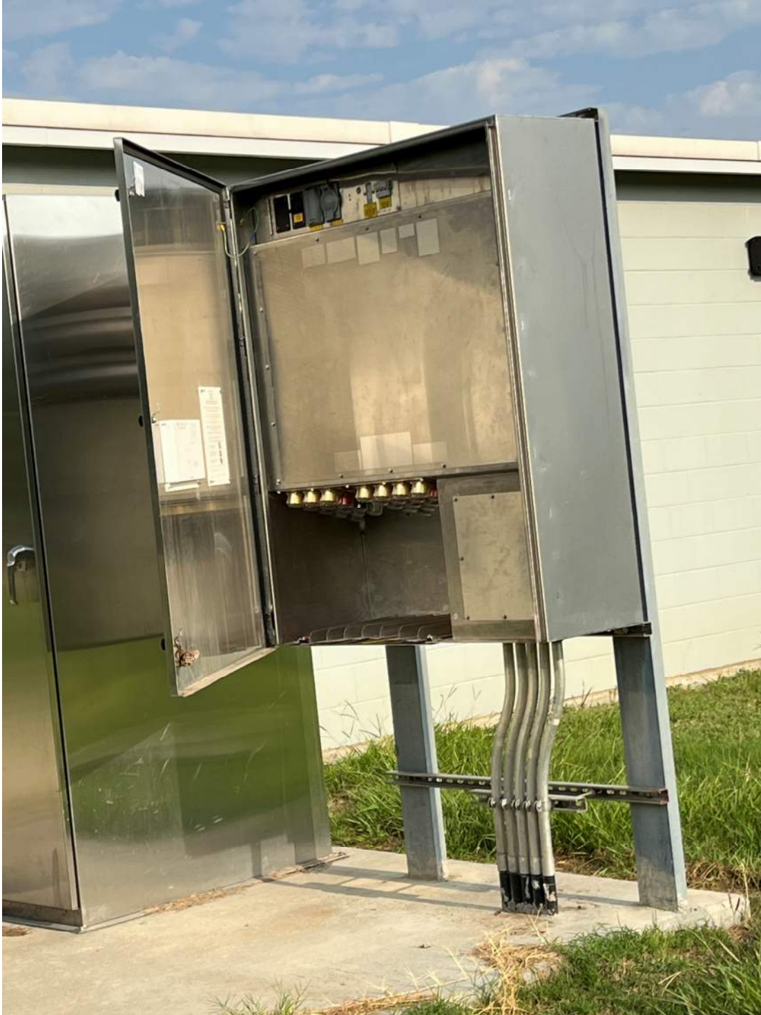
1. Existing Portable Generator Connection Cabinet (CAMLOCK)
