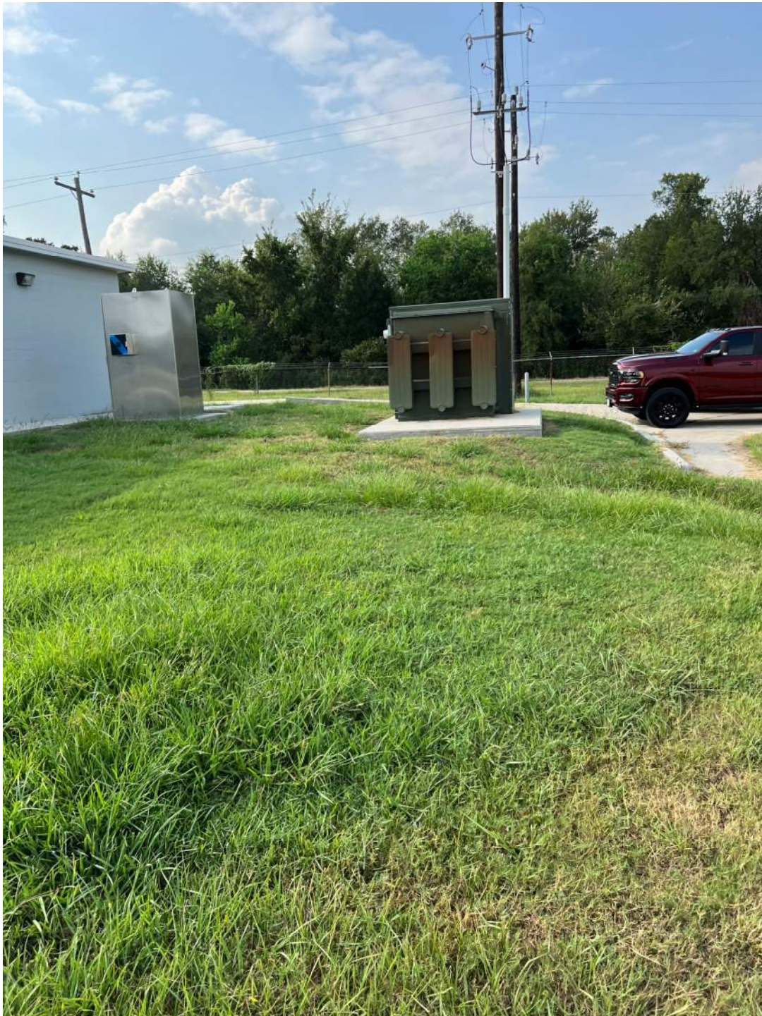
2. Existing Transformer and Gen Set Pull Box
